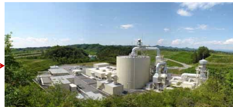
Hydrogen and Fuel Cell Vehicle Safety Evaluation Facility (Hy-SEF)
